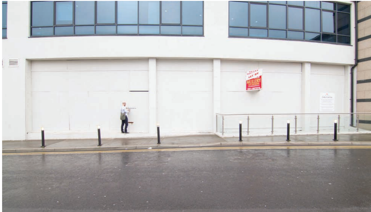
Street Frontage opening onto Station Road
