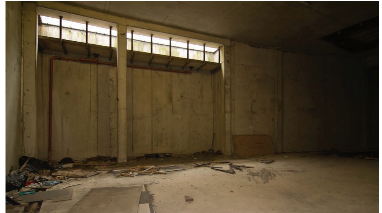
The Vault Space in the basement
